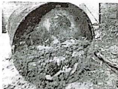
c) Leak proofing with mud
