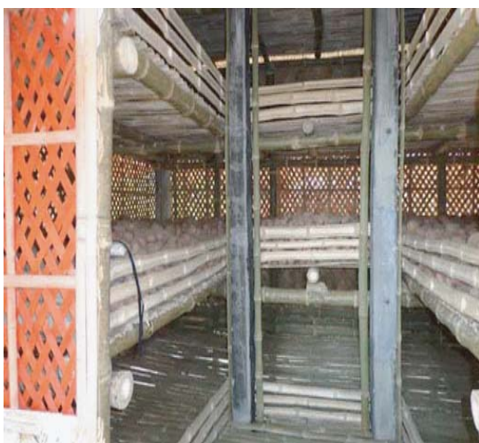
Fig. 3: Innovative potato storage structure (Reid et al. , 2011)
